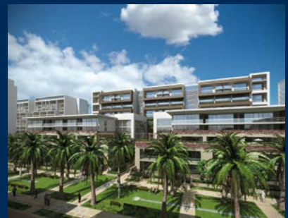
Al Zeina Housing Complex, United Arab Emirates
