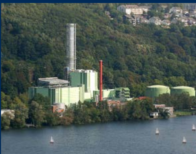
Gas Power Station Herdecke, Germany
