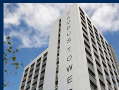
Hostel Campus Tower Magdeburg, Germany
